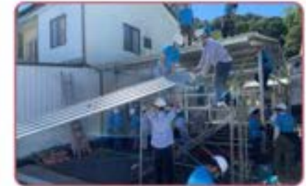
Construction of external walls/ roof steel structure
