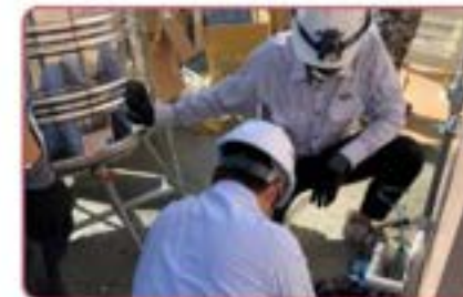
Installation of water pipes
