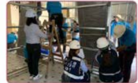
Installation of electrical circuit
