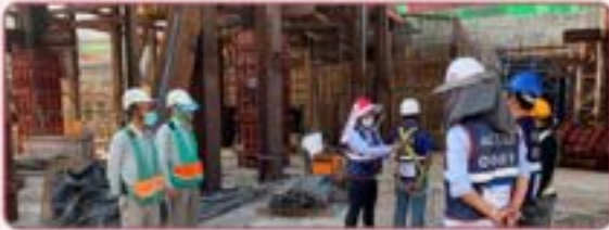
Emergency response education and training for contractors
