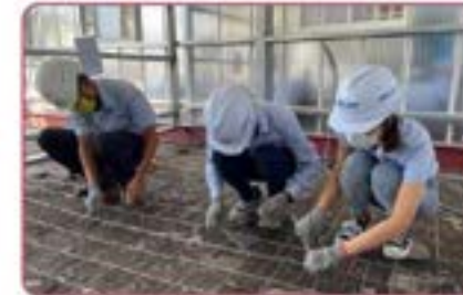
Foundation reinforcement with steel bars/ cementing
