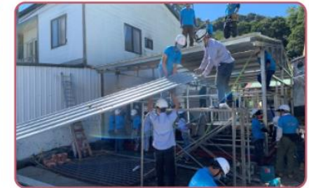
Construction of external walls/ roof steel structure
