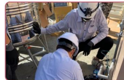
Installation of water pipes
