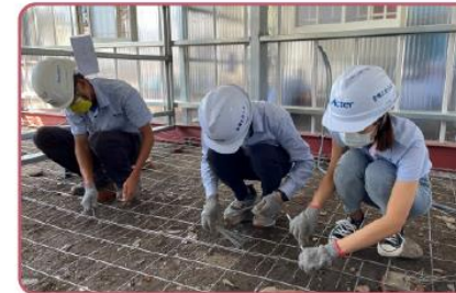
Foundation reinforcement with steel bars/ cementing
