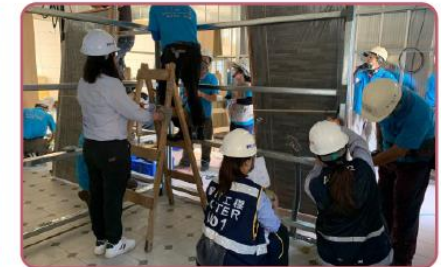
Installation of electrical circuit
